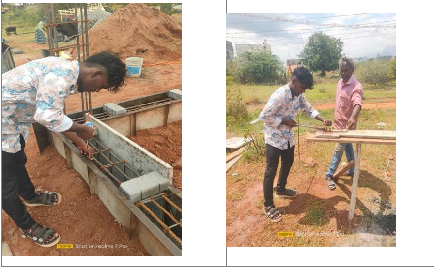
Fig 2.5.4 Reinforcement Detailing and Placement in Footing
